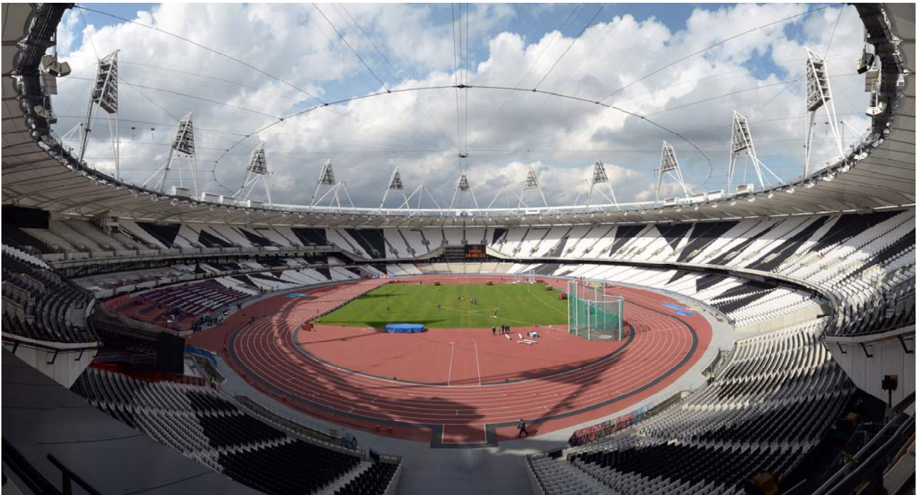
London 2012 Stadium, picture courtesy of London 2012
