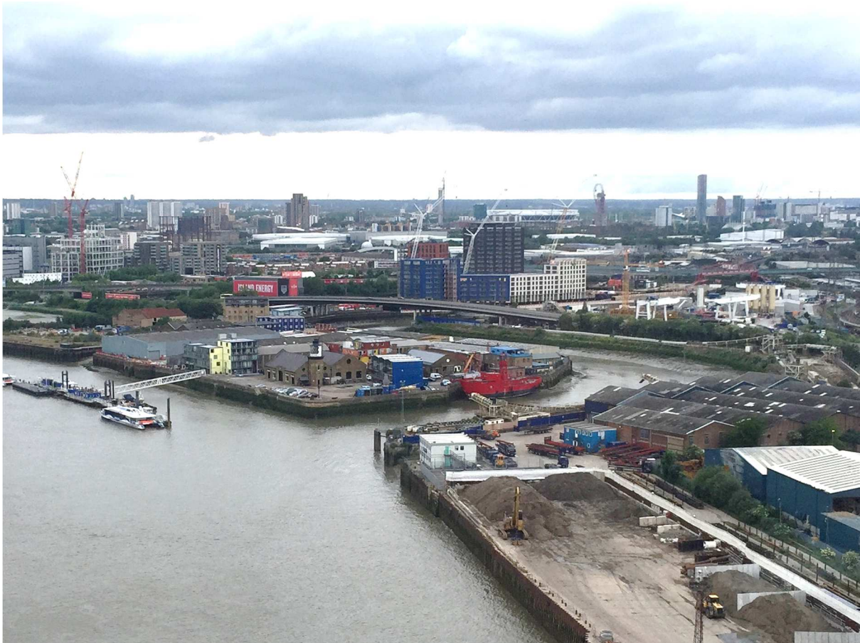
Aerial View of site from south east
