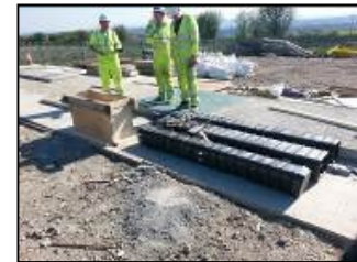
Fig. 1: Calder Bridge Trial
