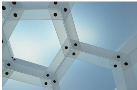
Figure 2: Close-up picture of pavilion and rivet connection details
