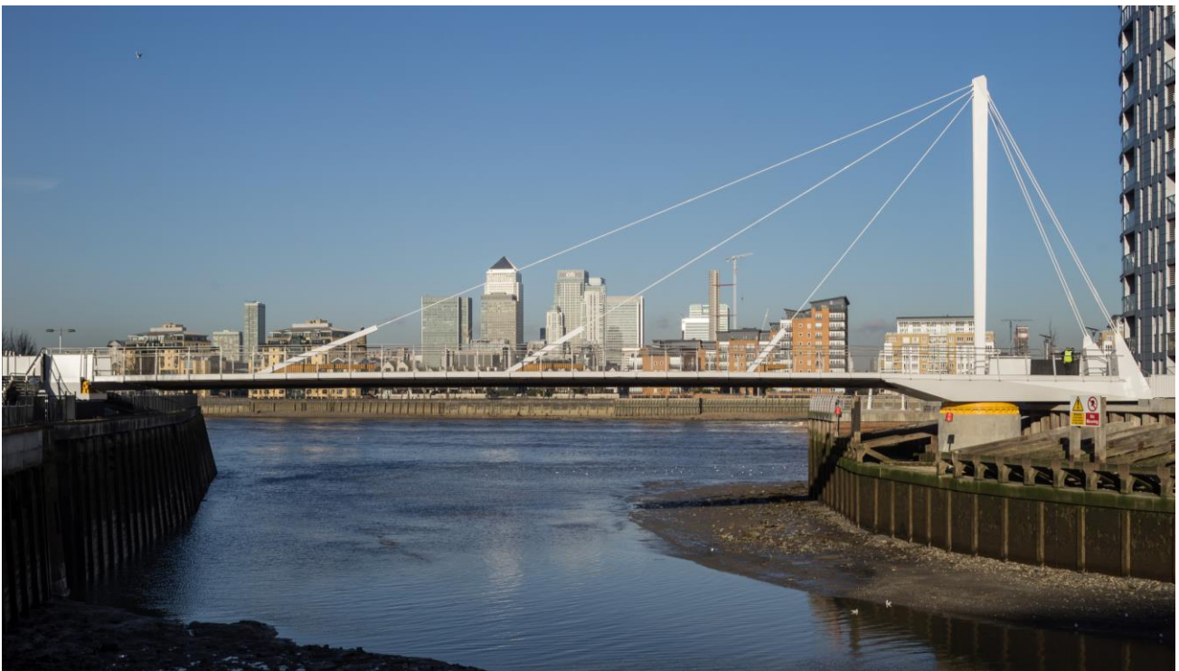
Greenwich Reach footbridge. Design: Flint & Neill with Moxon Architects and Eadon Consultants. Contractor: Raymond Brown Construction with SH Structures
