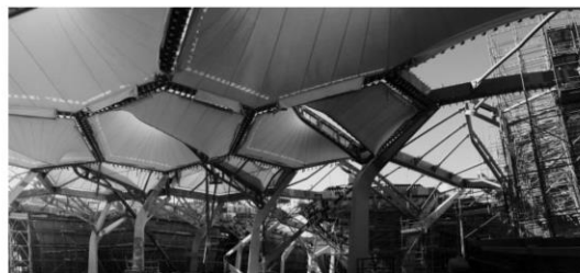
Fig.2: Some of the canopy cells during construction
