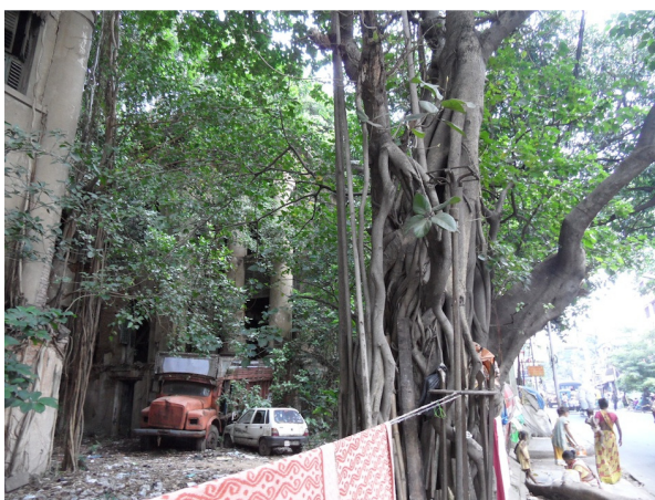
Two views of the building enveloped by a Bengal fig
