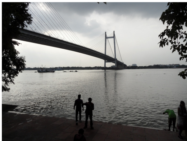
Second Hooghly Bridge
