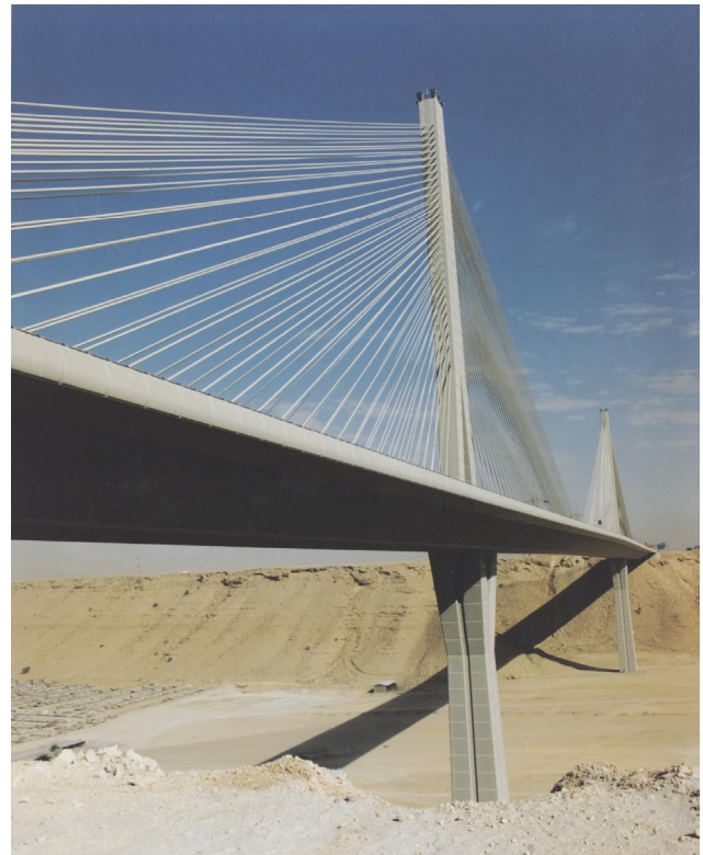
Wadi Leban Bridge, Saudi Arabia (Photos: Dar Consultants (UK) Ltd)
