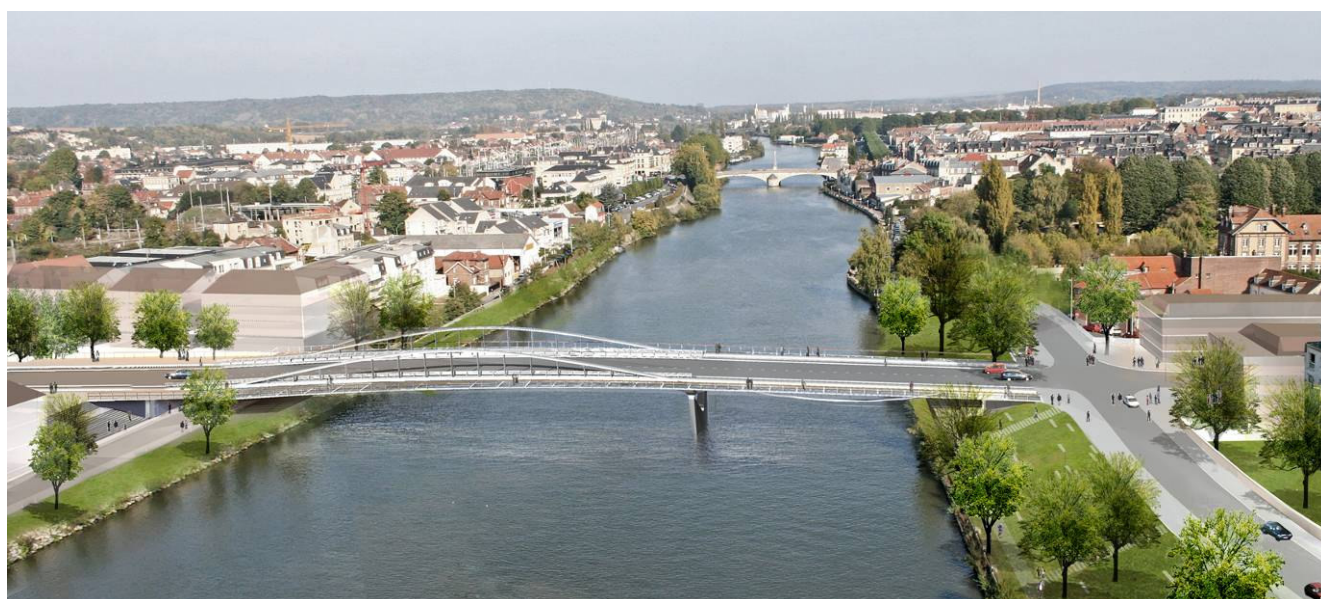
River Oise Bridge, Compiègne, France
