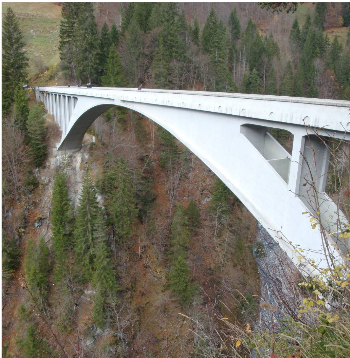
Salginatobel Bridge, Switzerland
