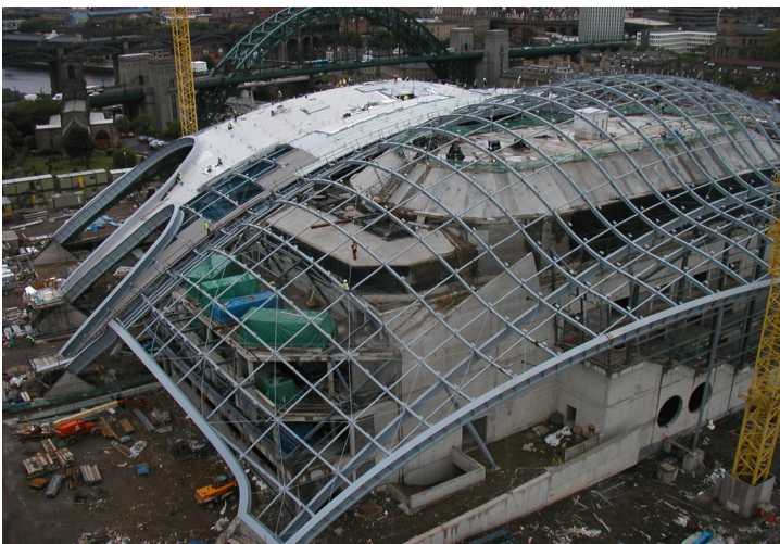
SAGE Music Centre Roof Enclosure, Gateshead, UK (during construction)
