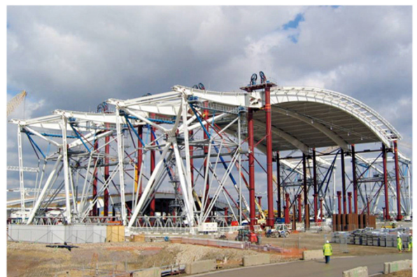
4. First section of the roof erected
