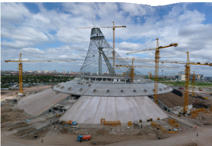
Khan Shatyr Entertainment Centre, Astana, Kazakhstan (during construction)
