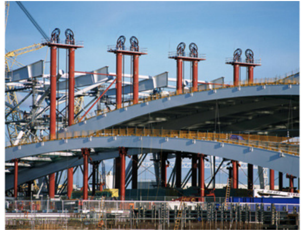
5. Roof under construction
