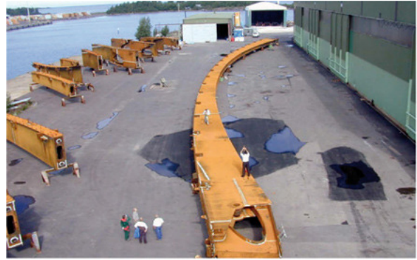
12. Rafter trial assembly and tolerance check
