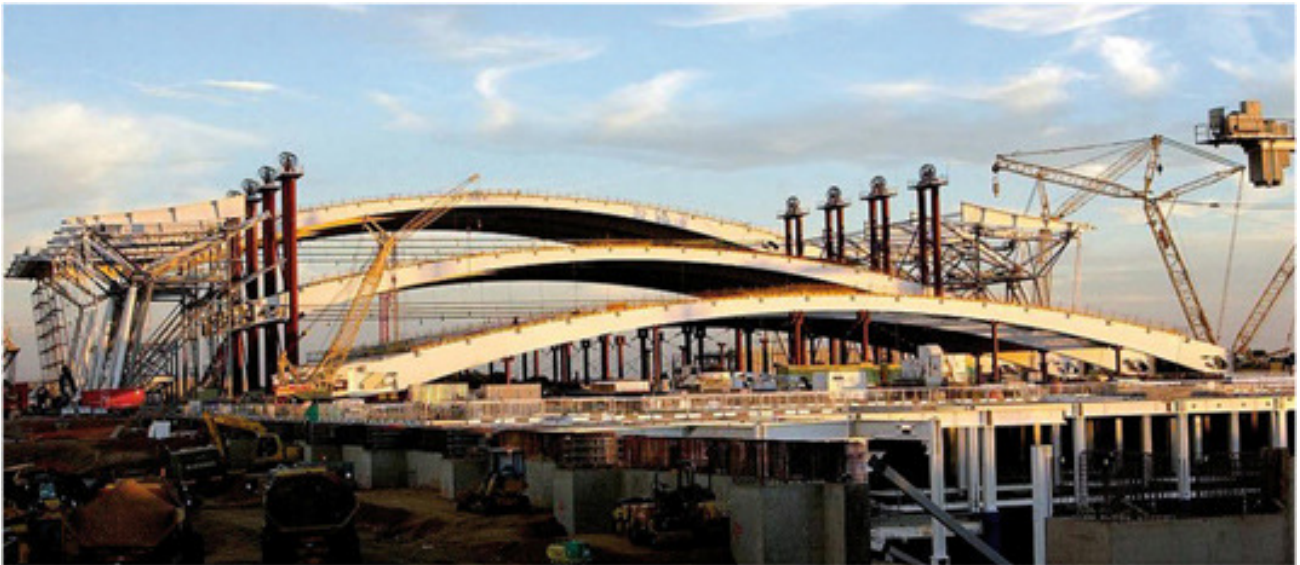
13. Roof structure under construction, furthest section complete, central section being jacked, near section assembled ready for lifting.
