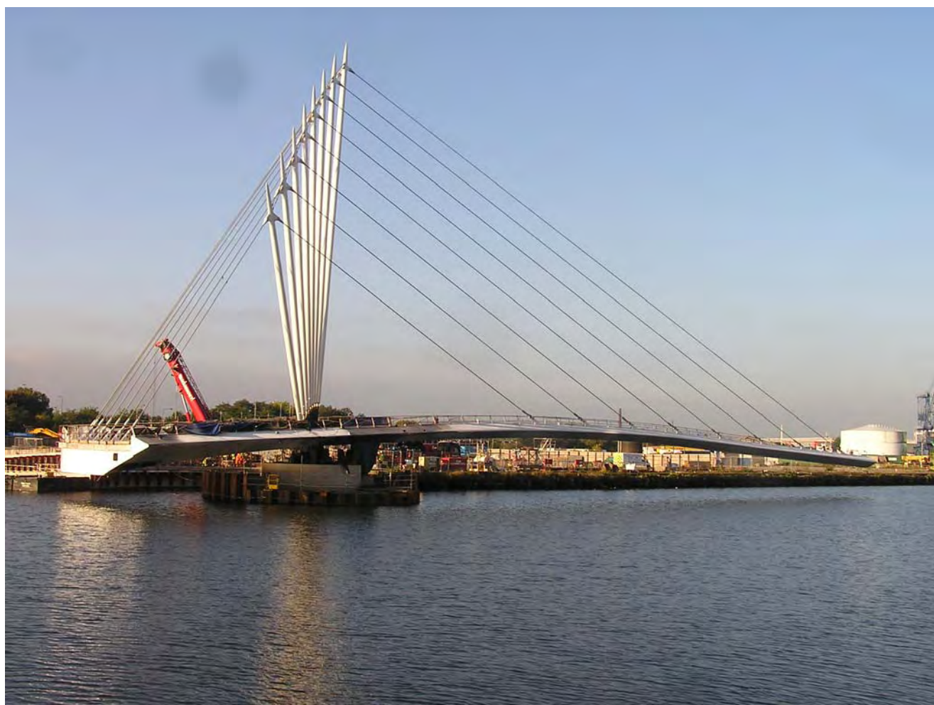
Media City Footbridge under construction, Salford Quays, October 2010
