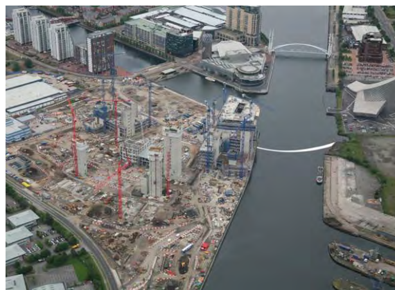
Aerial view of footbridge location
