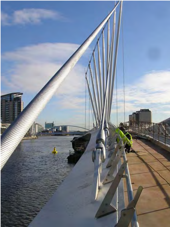
Footbridge under construction, October 2010
