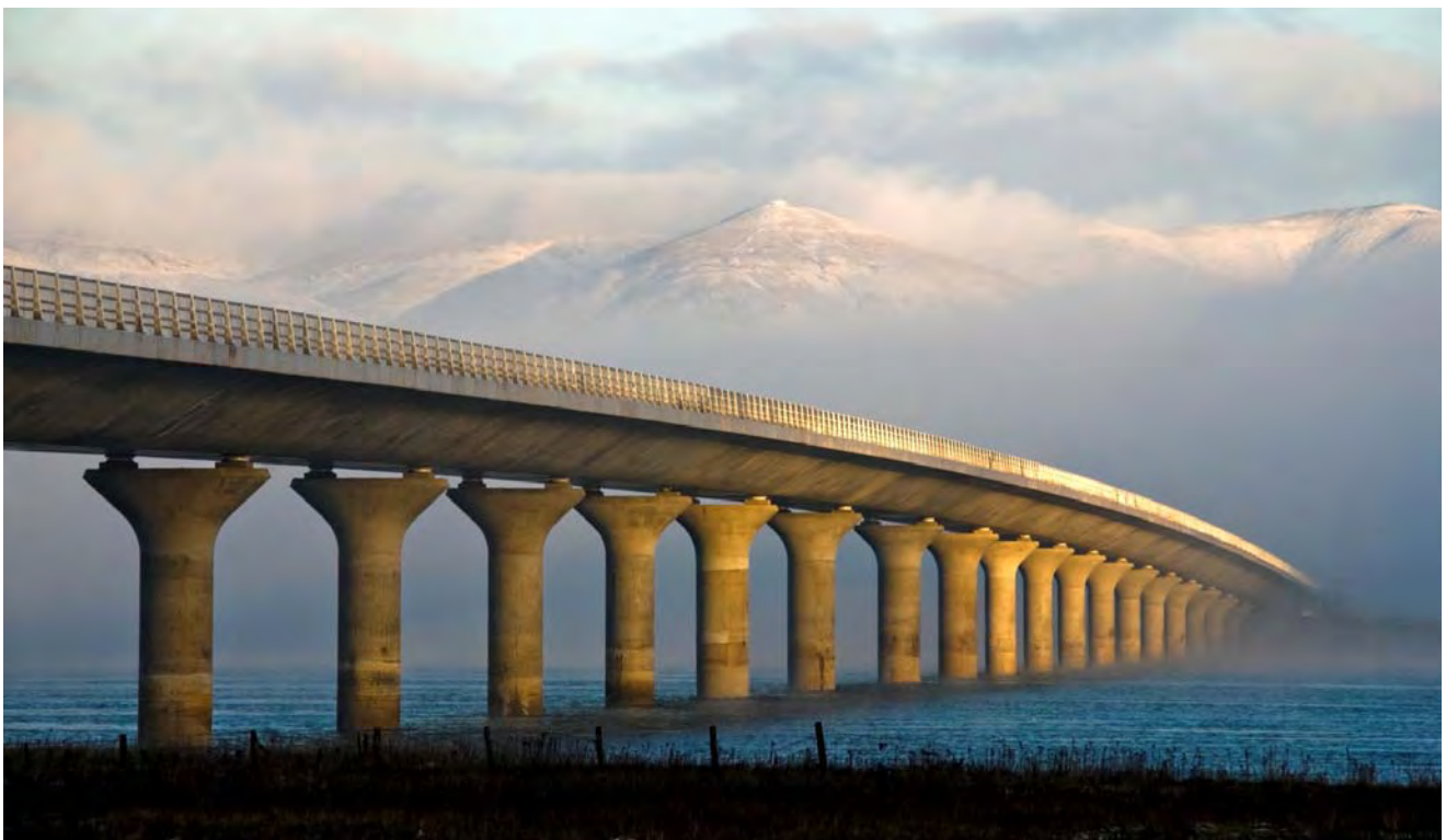
Clackmannanshire Bridge, design by Simon Bourne with Benaim
