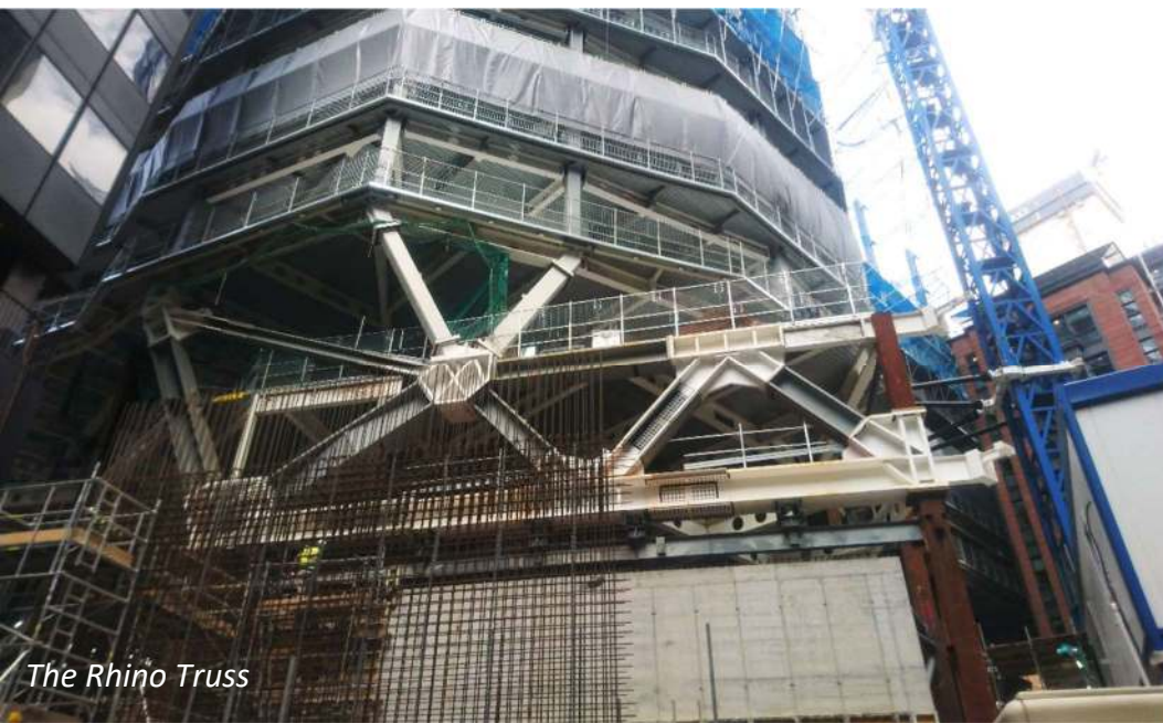
Top-Down construction 20 levels of core; no foundations
