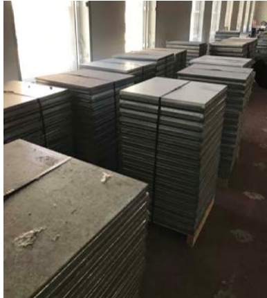
Raised access floor tiles deconstructed and grouped to be sent for reconditioning before being reinstalled in office building.
