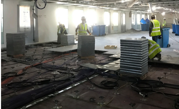
Raised access floor tiles deconstructed and grouped to be sent for reconditioning before being reinstalled in office building.
