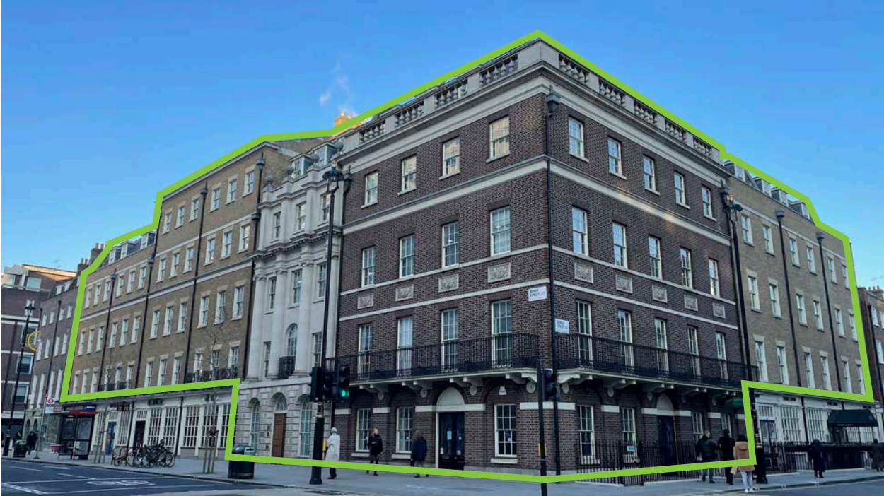
Existing External View of Office Building
