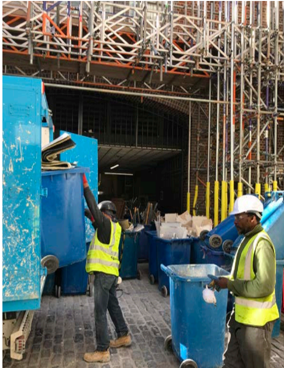
Removal of reuse material to be sorted
