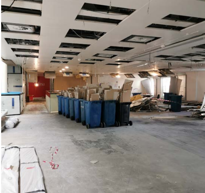
Soft strip out of ceilings
