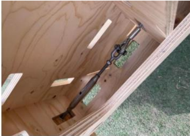
Fig. 10 Cable within block to provide tensile capacity at bottom of the beam
