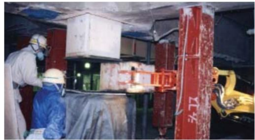
Figure 9. Cutting Columns © Kajima
