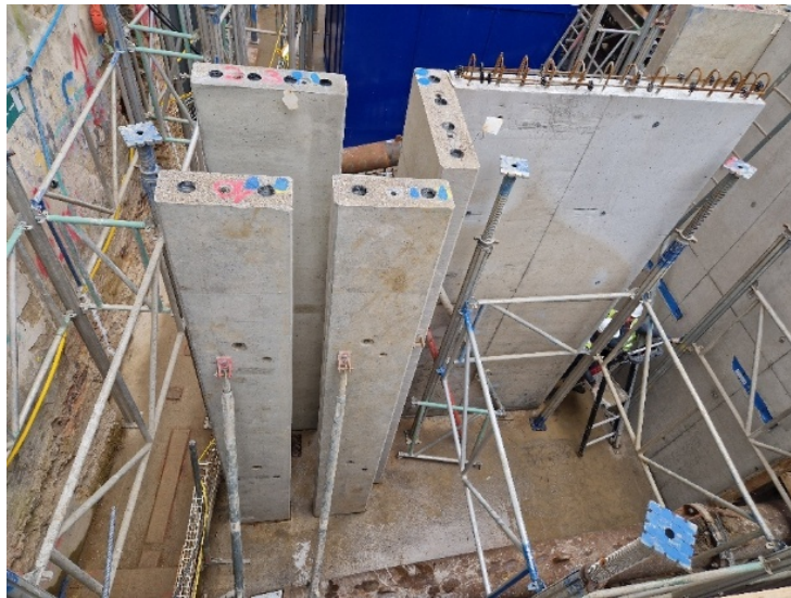
Figure 4: Core construction in progress on site, precast columns with dowel holes in top, in-situ wall with exposed reinforcement to right
