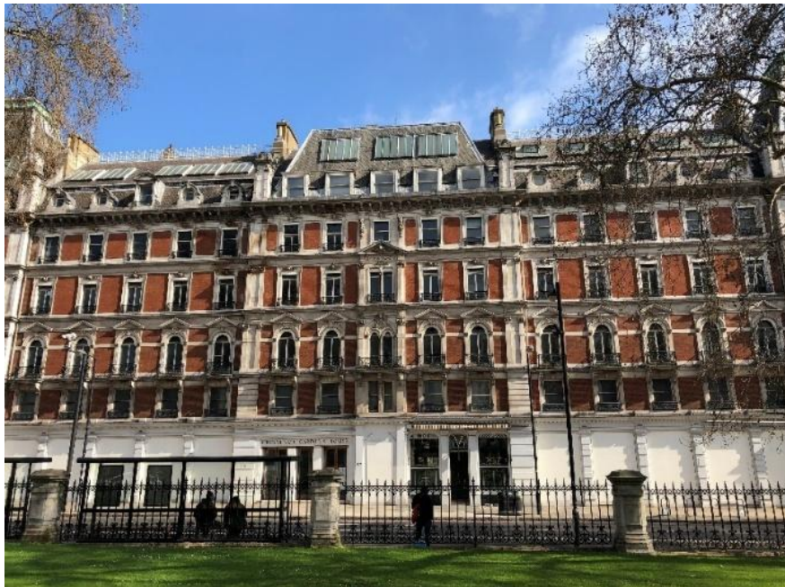
Figure 1: Looking north to Grosvenor Gardens House, 2021
