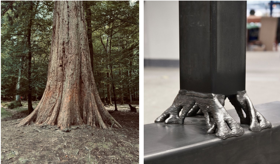
Topology-optimised hybrid node resembling the branching form of a tree root
