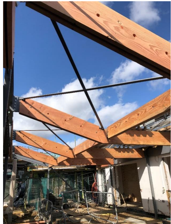
Figure 6 - Site Progress Photo
