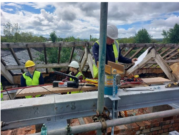
Figure 7 Temporary jacking arrangement
