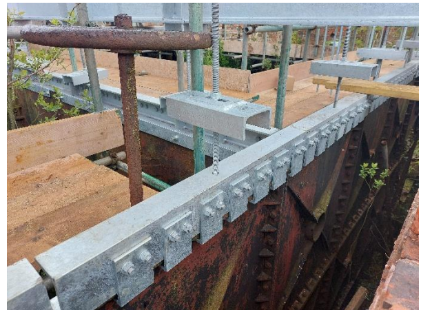
Figure 5 Clamps installed to the tank walls
