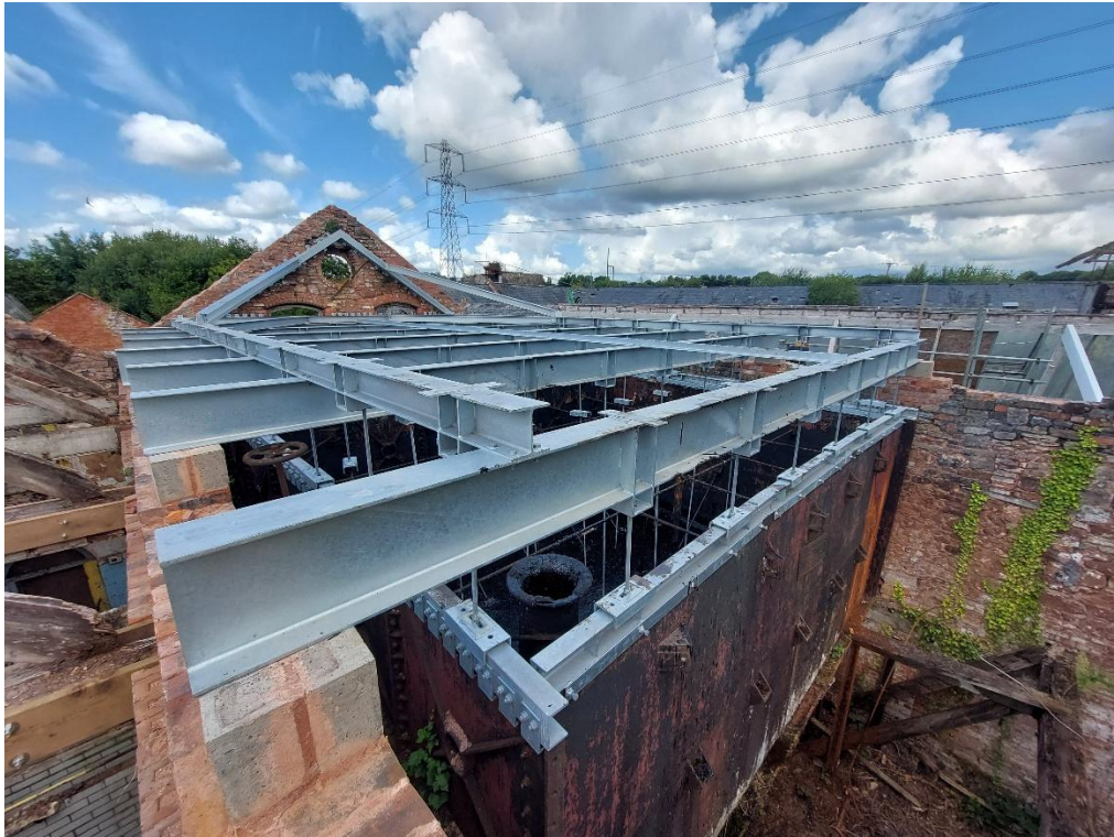
Figure 9 The completed structure
