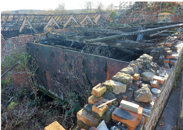
Figure 2 The adjacent buildings provided limited access
