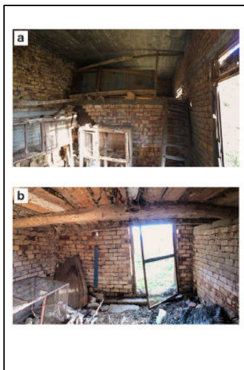
Fig. 2a-b: Existing interior and low timber mezzanine.
