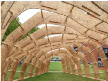
In a pro bono effort, a small team of young engineers at Arup collaborated with the artiste to design and explore the form of the unusual and highly surprising structure. Using plywood-like material to build such a structure is unusual and standard building codes were inadequate to design such complex, curved beams. Due to the low self-weight and sensitivity to wind action, an advanced numerical approach was taken to analyse the behaviour of this deceptively complex structure.
