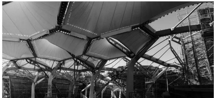
*Fig.2: Some of the canopy cells during construction*
